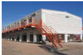
Local Equipment Rooms
