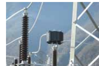
Installation of line traps
